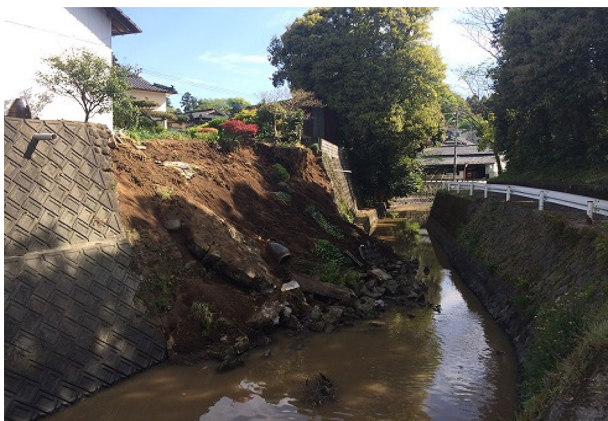
Fig. 10 Example of collapsed irrigation channel in the Shirakawa River Basin
